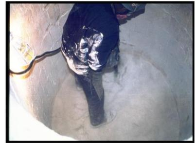
The worker enters the confined space of the furnace to ram loose silica until the surface is solidly knit. Depending on the size of the furnace, this activity can be lengthy, exceeding one hour, exposing workers to airborne dust and repetitive-strain injury.
